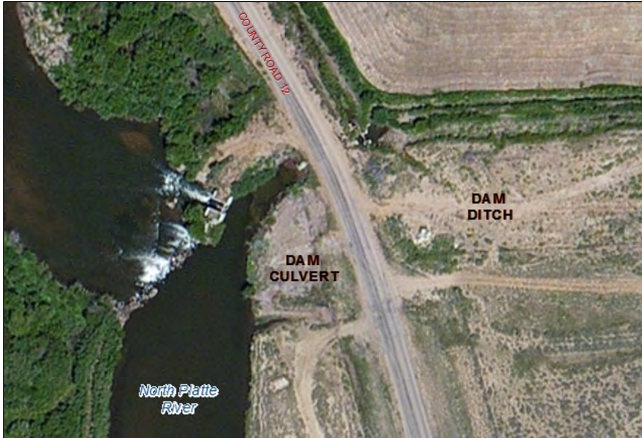
Figure 35. Ditch Dam Headgate Improvement Project
